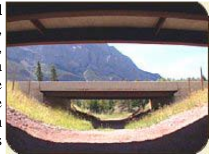
Underpass proven highly successful for moose crossing beneath railroads or roads
